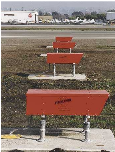
PAPI Precision Approach Path Indicator
