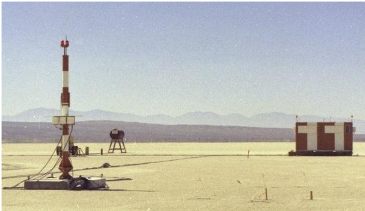
Mikrowellen-Landesystem (Microwave Scan Beam Landing System, MSBLS)
